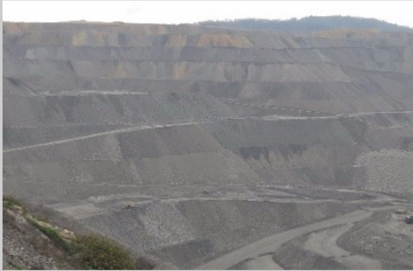
Very high spoil dumps at Mt Owen mine.
